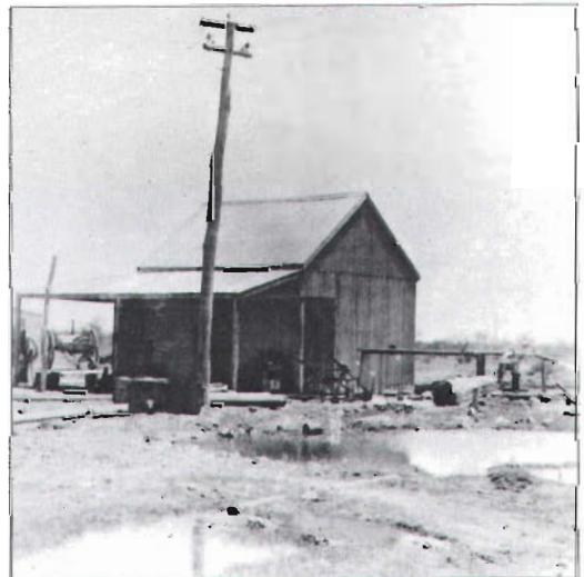
Thargomindah Power Station
