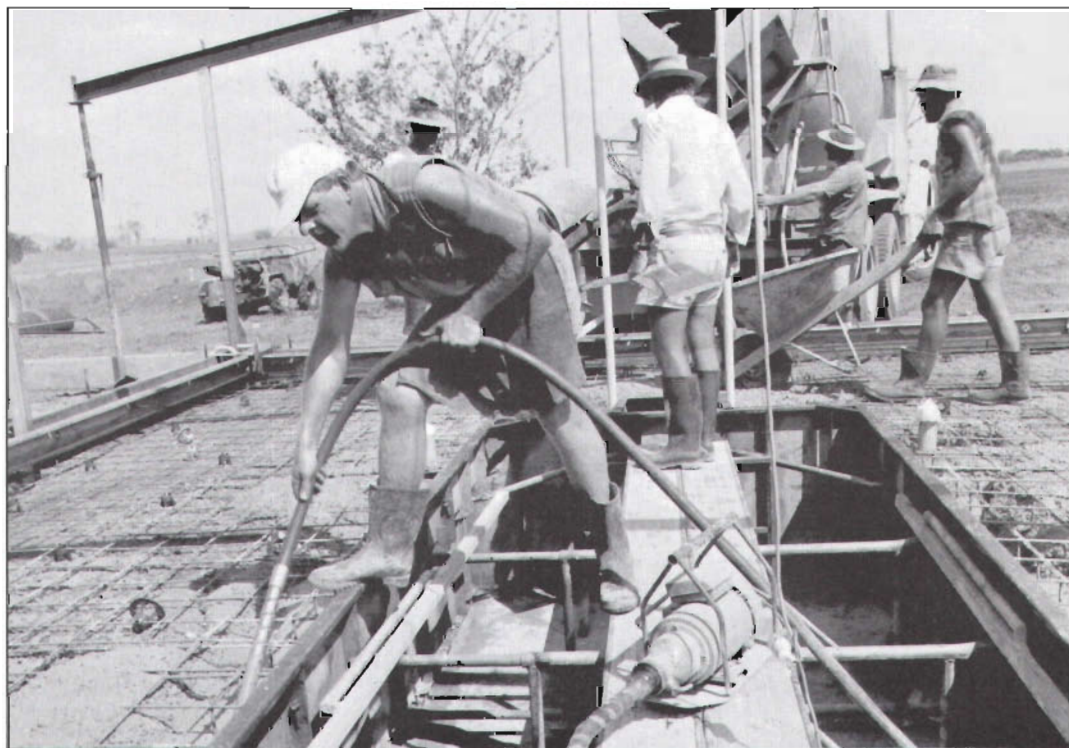
Concreting a dairy, Pecks Crossing
