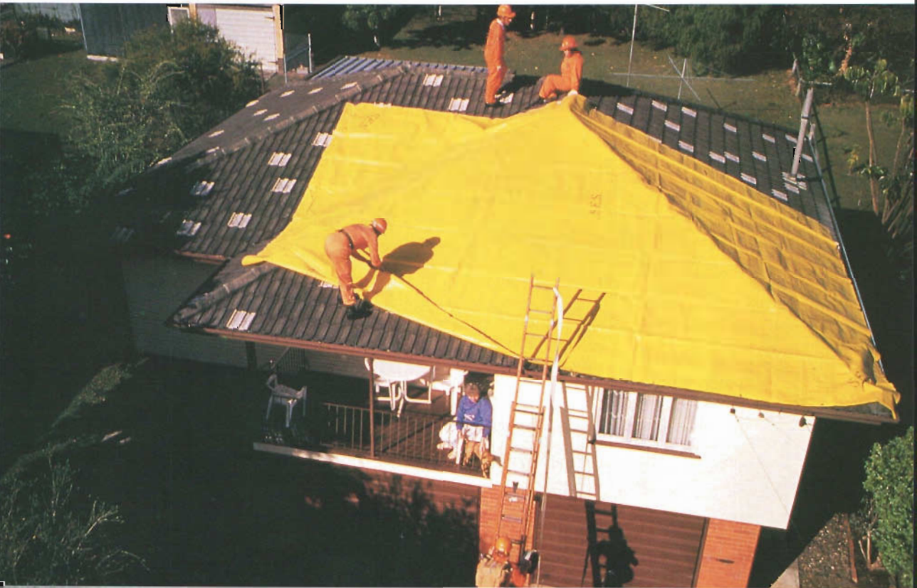
Tarpaulin laying practice
